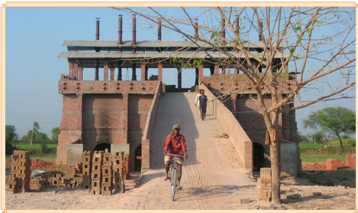
A vertical shaft brick kiln
