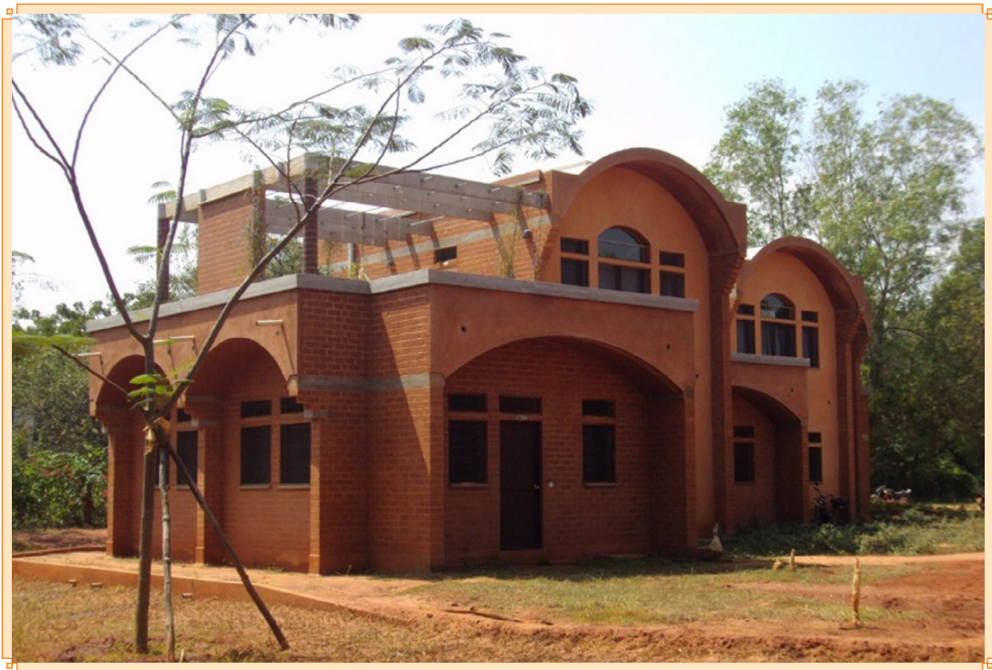
A building constructed using LC 3 at the TARAGram Campus in Orchha, Madhya Pradesh.
