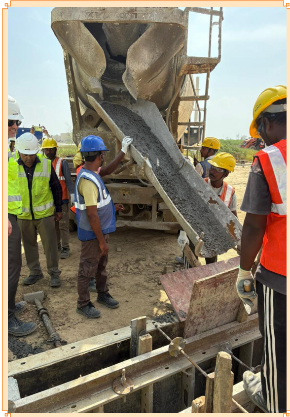
Adoption of alternative materials in an on-site construction site
