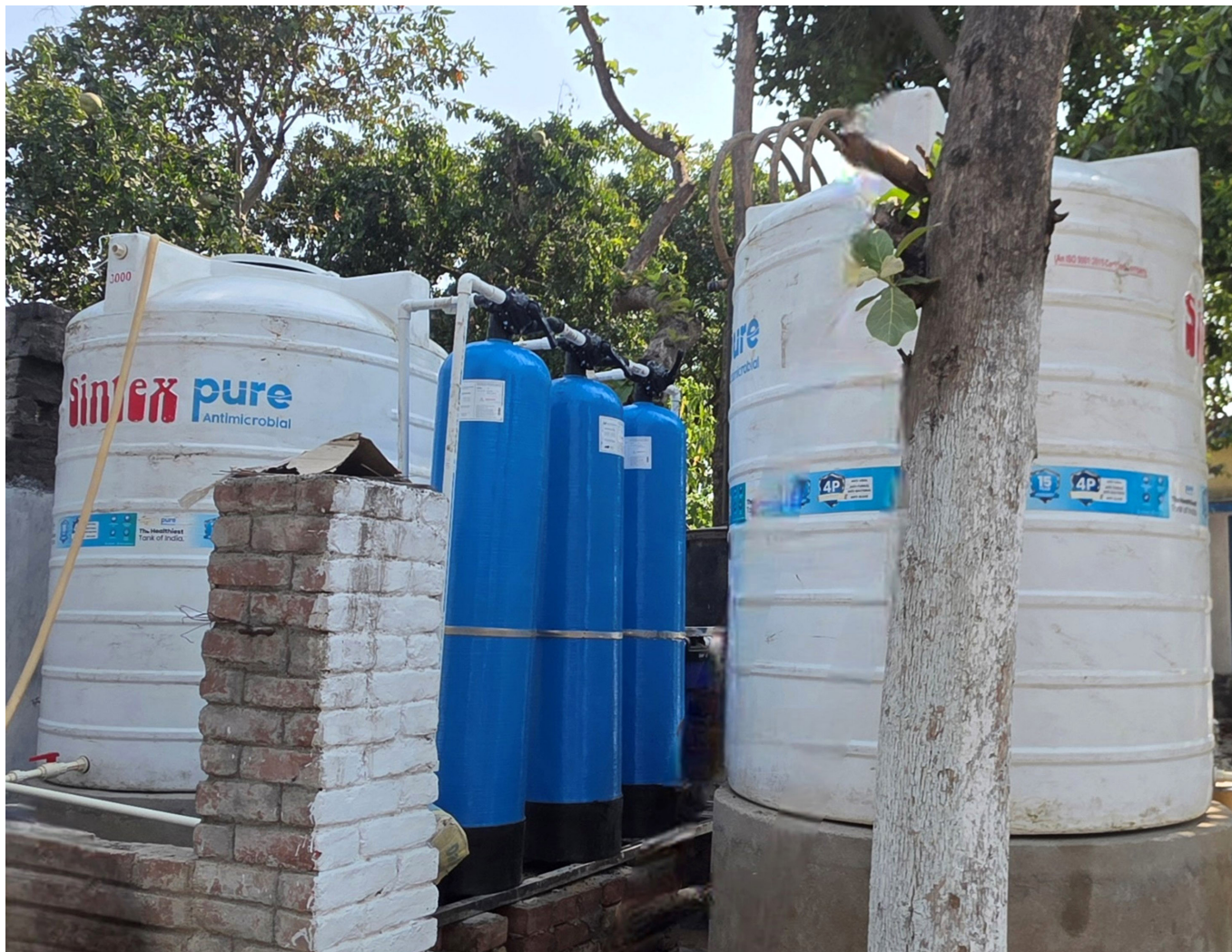
Arsenic removal filters installed in the village
