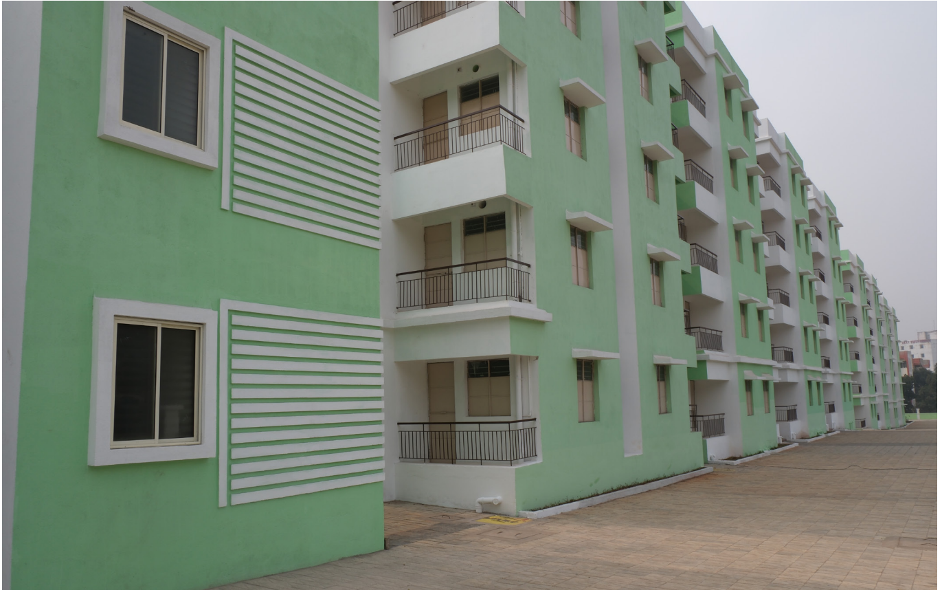
Residential structure with G+4 stories completed by BDA, Adjacent to N.H-16, Kalinga Nagar Zone K-9 (B)
