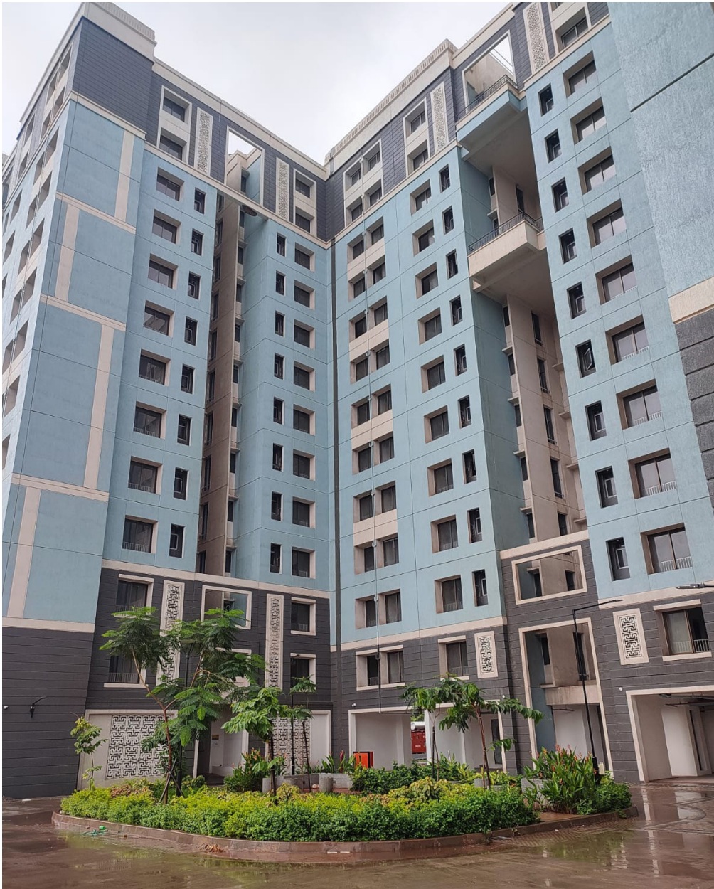
Affordable housing project with precast RCC wall panels and precast roofing slab, at Kharkopar, Navi Mumbai, constructed by L&T
