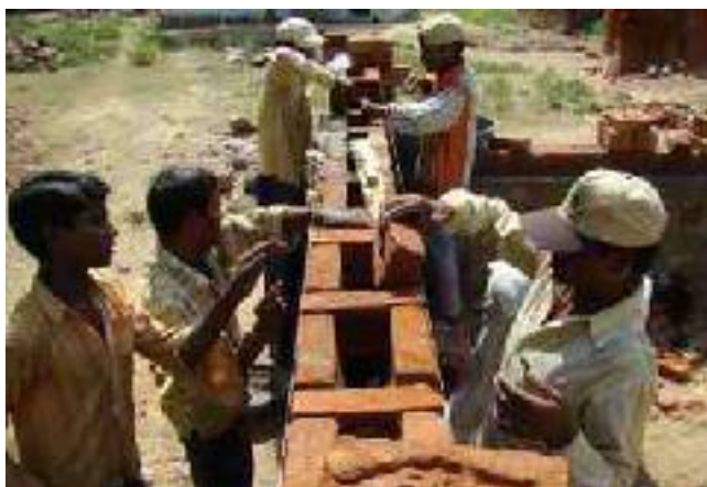
Trained masons at work
