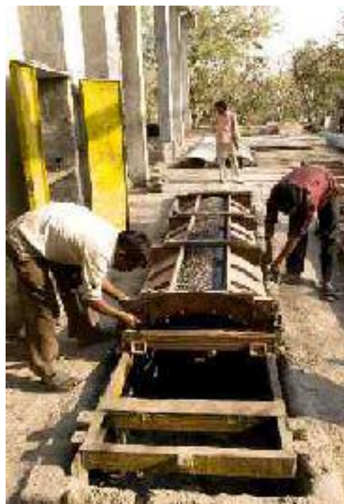
Community workers manufacturing roofing channels
