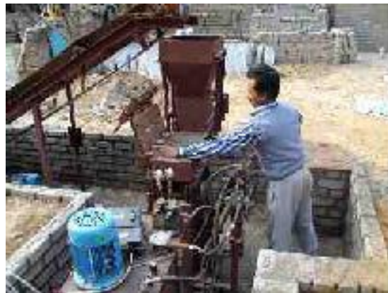
A brick making enterprise
