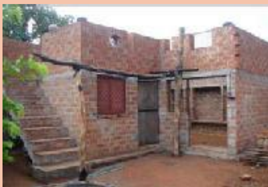
Construction of Eco House
