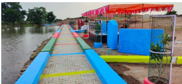
Walking track constructed around the pond
