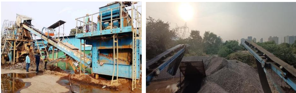
C&D Waste plant at Daigarh, Thane
