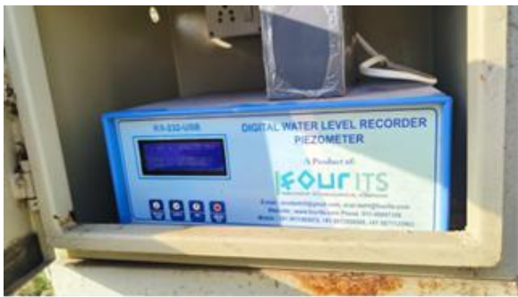
Piezometer installed at pond site in Mojabad
