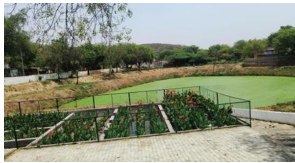
Hariahera pond STP is installed at site that uses root zone technology to treat sewage water
