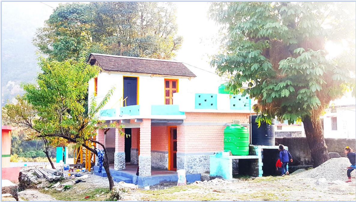
Installed Jal TARA water filter at community building in Kamad village, Uttarkashi
