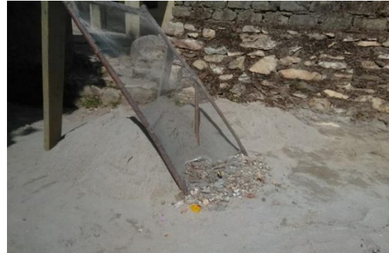
Sieving process of sand
