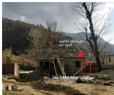
The selected site at one of the community building in Kamad village, Uttarkashi to install the water system.
