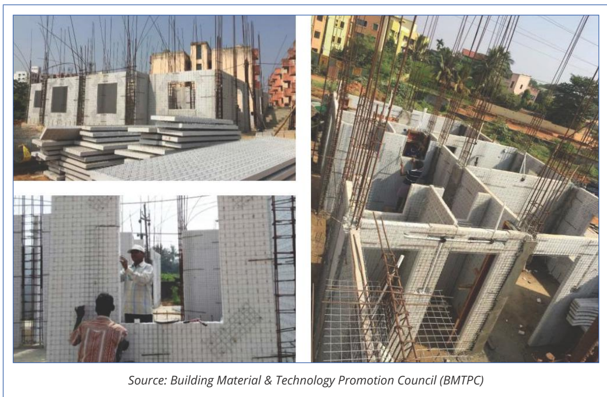
Figure 10: Prefabricated construction – EWS housing in Chandrashekharpur
