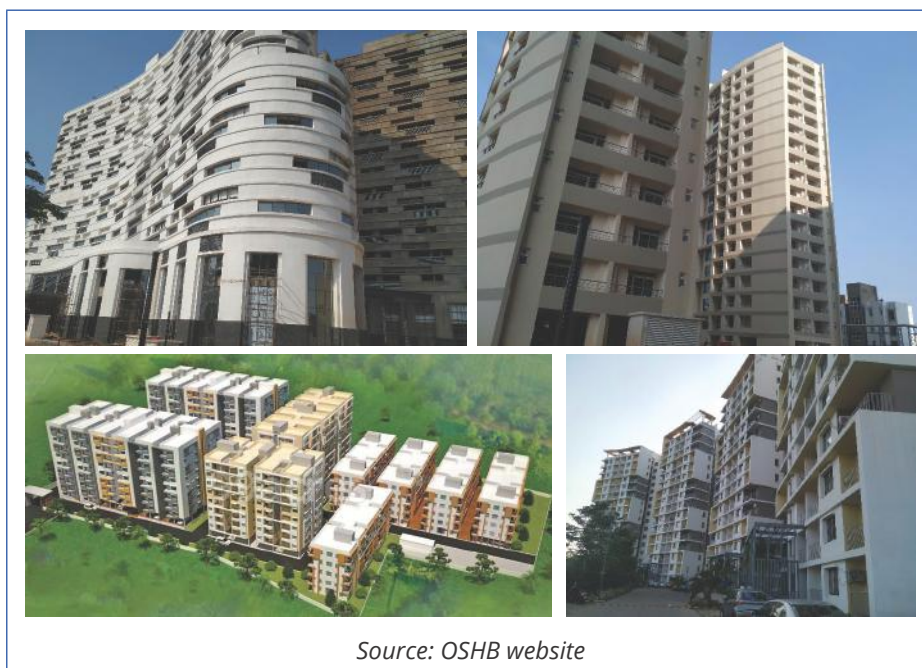
Figure 7: High rise residential construction in Bhubaneswar
