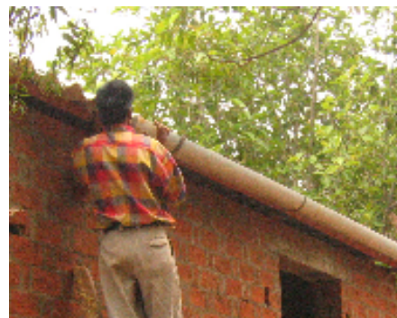
Setting up RWH at slanting roofs
