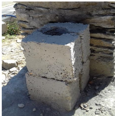
Overlapping of hollow concrete blocks.
