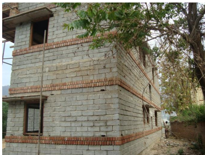
Residential building using concrete block in Srinagar, Uttarakhand
