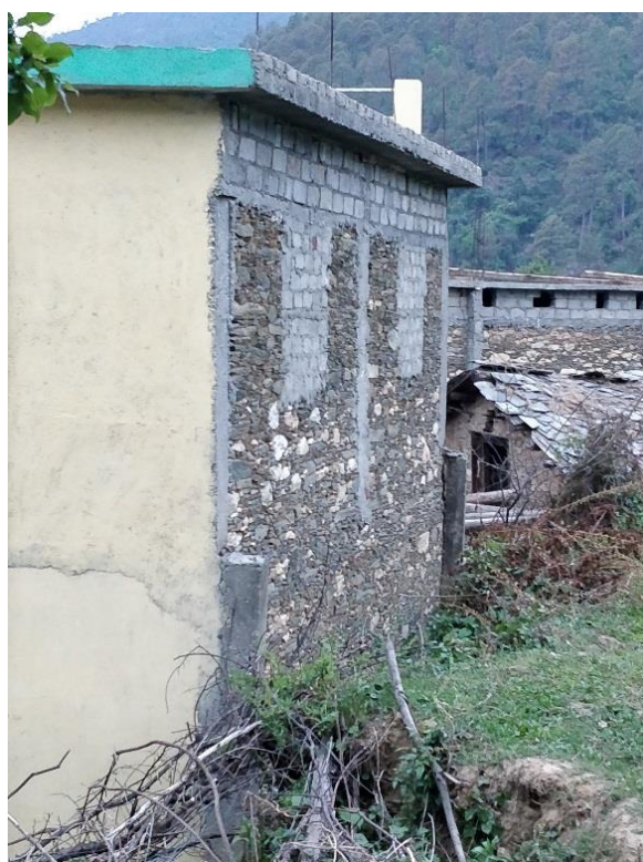
The use of concrete blocks as a filler in stone wall masonry at Thandi village, Uttarkashi
