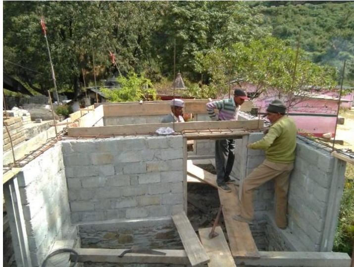
Double storey concrete block structure in community building at Kamad village, Uttarkashi.
