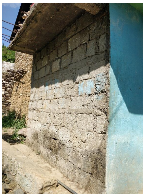
The concrete block masonry with direct load of RCC slab on it at Kamad village, Uttarkashi
