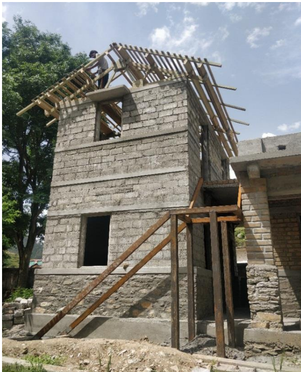
Ground floor masonry and complete double storey masonry with concrete block in community building at kamad village, Uttarkashi.
