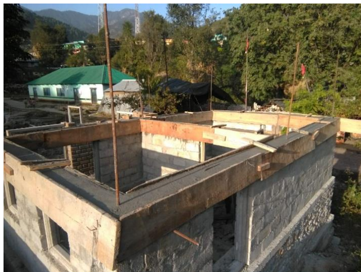
Double storey concrete block structure in community building at Kamad village, Uttarkashi after external finishes with lime plaster and paint. Lintel band casting over concrete block masonry.
