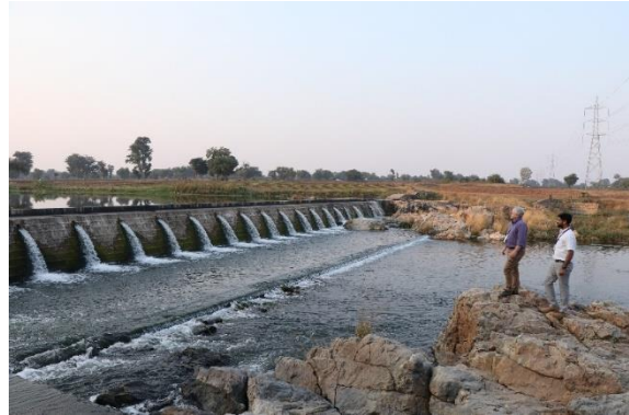
Field visit to the Gurari Check Dam near Orchha
