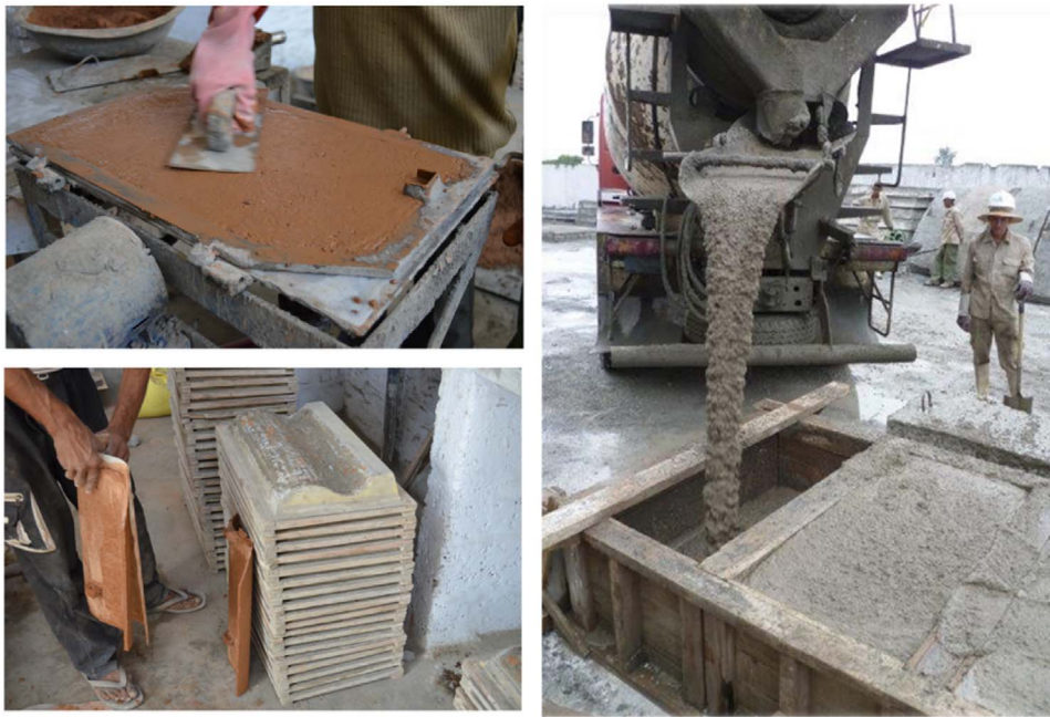
Fig. 3. Examples of application of LC 3 : micro-concrete roof tiles in India (left) and precast concrete blocks in Cuba (right).
