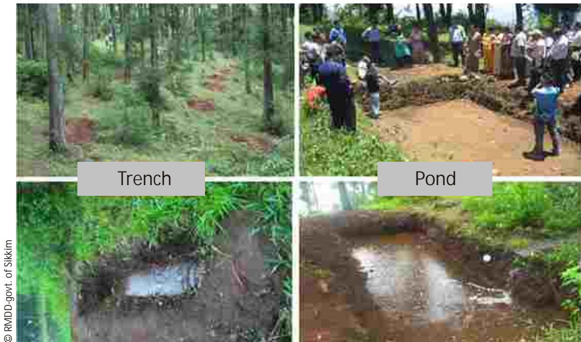
Water harvesting structures
