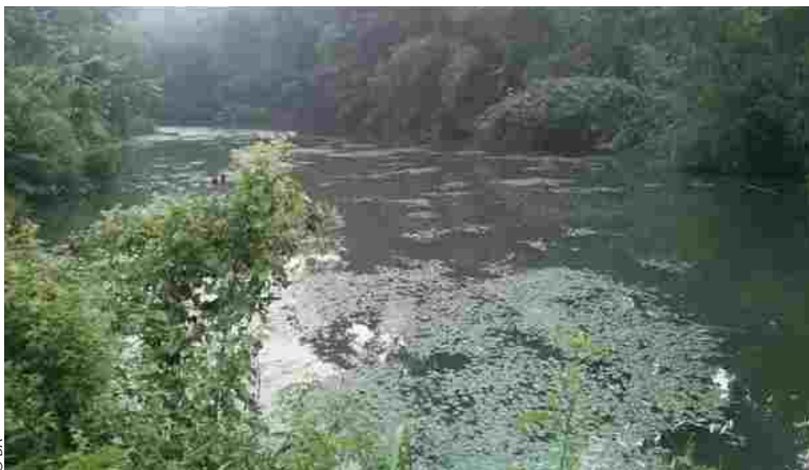
Checkdam reservoir also used for fishery
